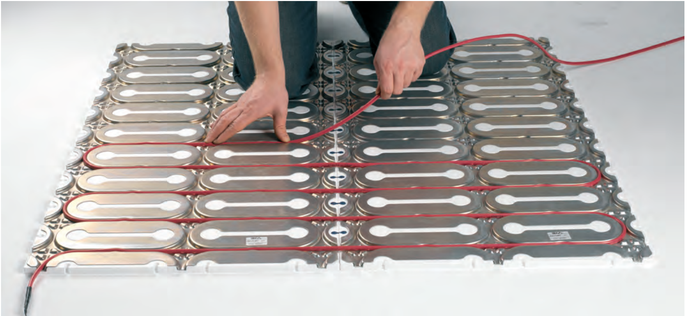
Fig. 20. Mounting method for heating cable into DEVIcell™
