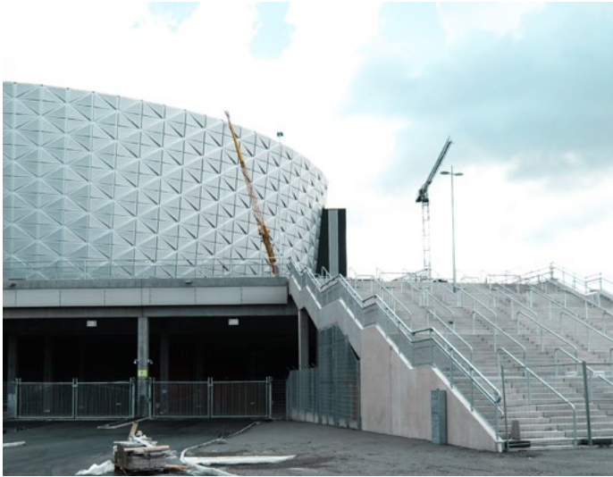
Cable distribution cabinet at the construction of the "Friends" Arena in Solna, Sweden.
