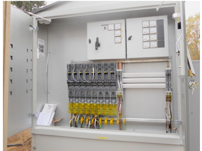
Kabeldon switching devices SLDL, Sweden, especially designed for CSS.
