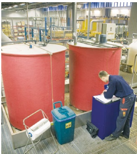
Treatment for outgoing waste water from surface treatment.
