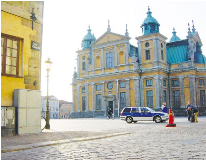
Distribution board, Kalmar, Sweden.
