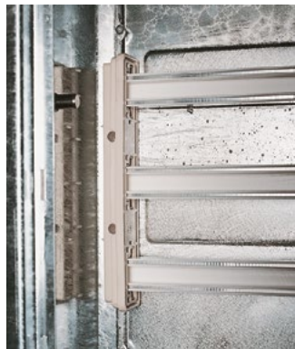
Sliding busbar counteracts damages from frost heave.
