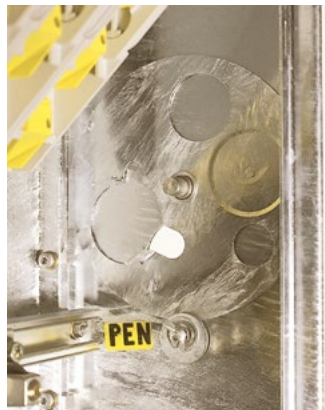
Temporary openings at both sides of the enclosures.
